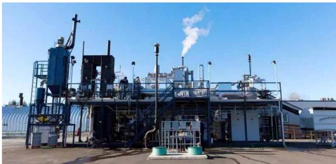
Janicki Omni Processor能将干燥的粪便和污泥转化为热能和电力
